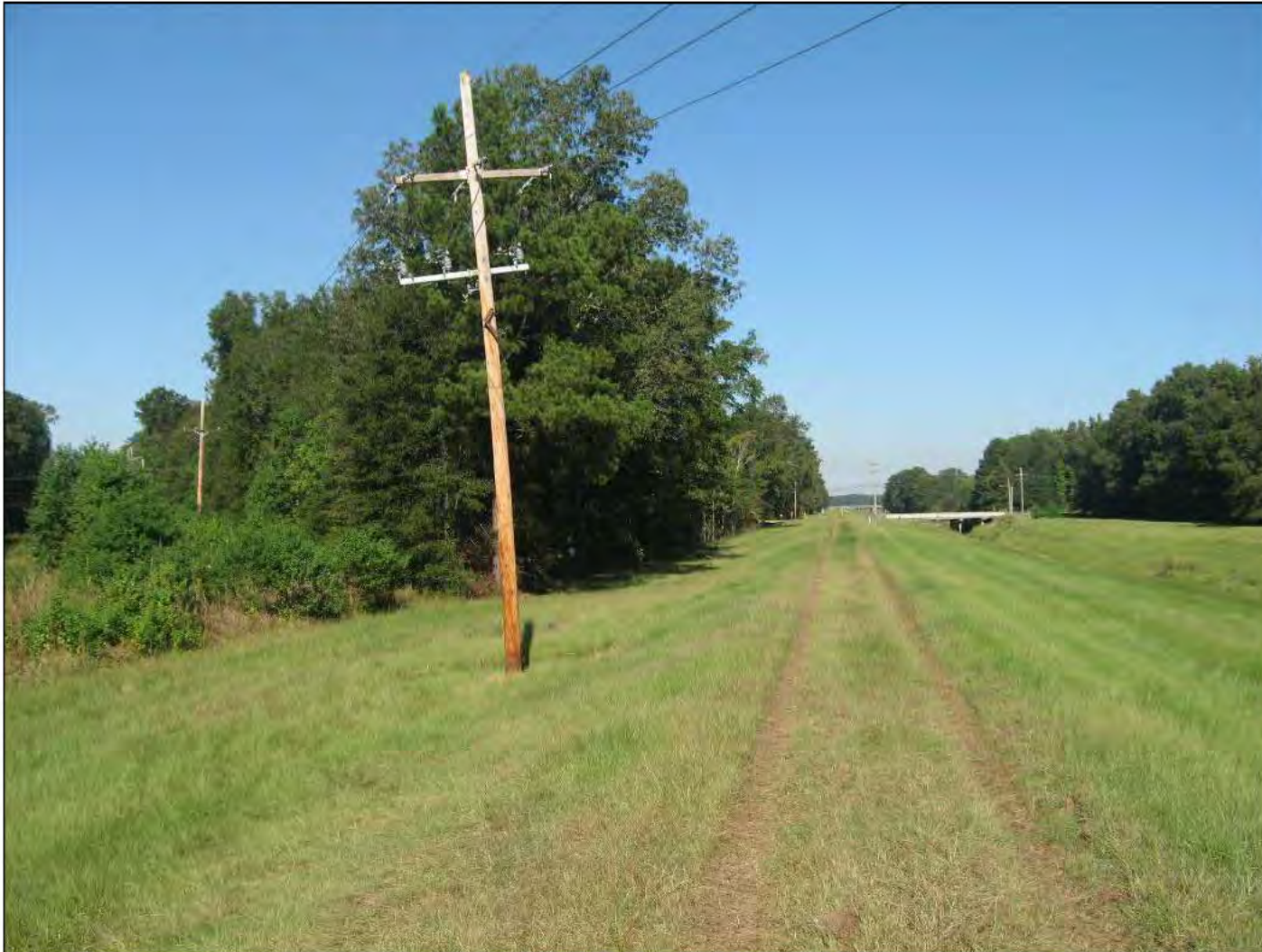
Inspect ID: EJFC_2016_a_0004 Title: USACE_CEMVK_EJFC_2016_a_0004_1.jpg Rated Item: 3. Encroachments Caption: Rating: Minimally Acceptable; Remarks: STA 36 LS utility pole; Station_1: 36
