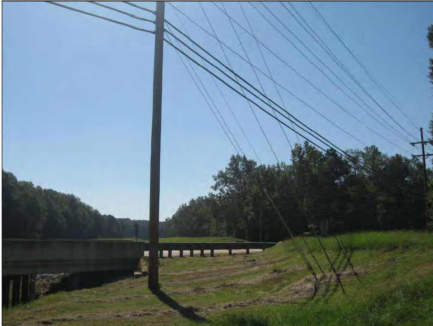
Inspect ID: EJFC_2016_a_0006 Title: USACE_CEMVK_EJFC_2016_a_0006_1.jpg Rated Item: 3. Encroachments Caption: Rating: Minimally Acceptable; Remarks: STA 46 RS and LS Utility poles on either side of Mangum Dr. scheduled to be removed ; Station_1: 46
