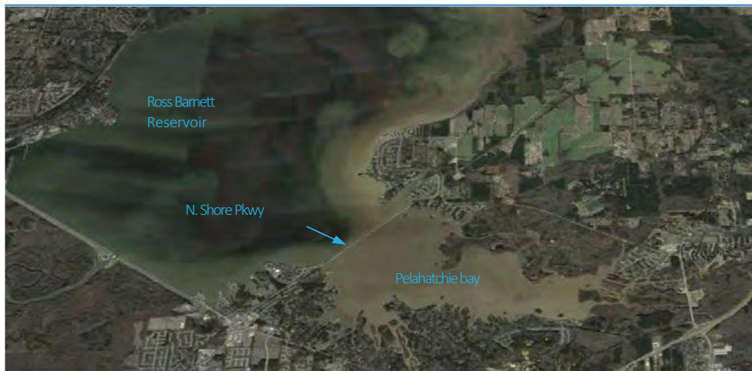
Figure 5. Aerial visual (2020) of sedimentation in Pelahatchie Bay from construction activities.
