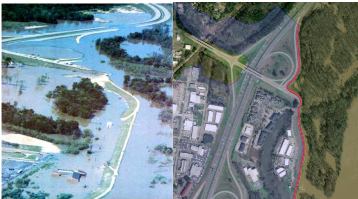
Figure. 2-7. 1984 Levee Extension to Prevent Flanking
