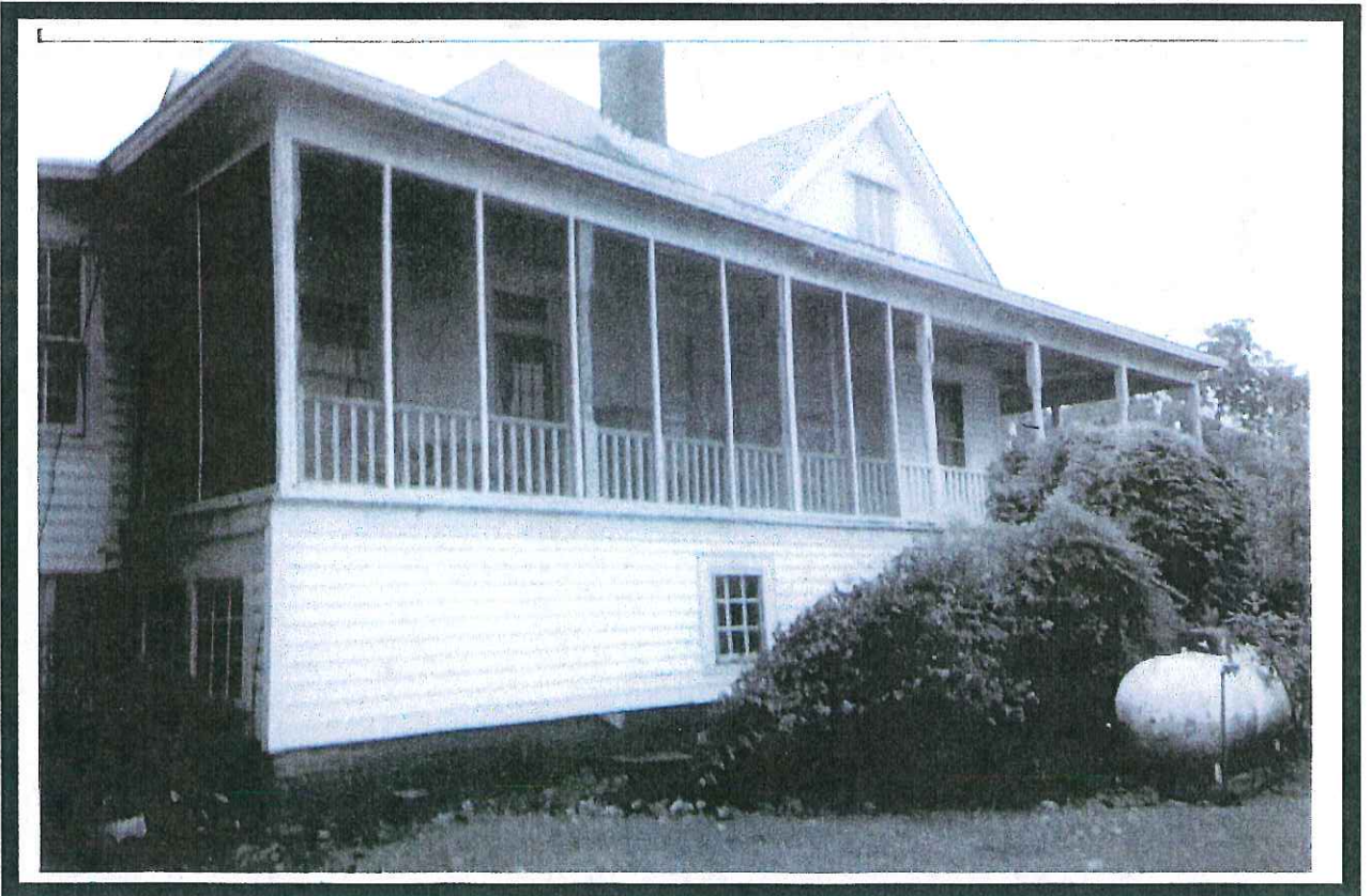
Figure 304. Legette Farm; a. view west; b. view east.
