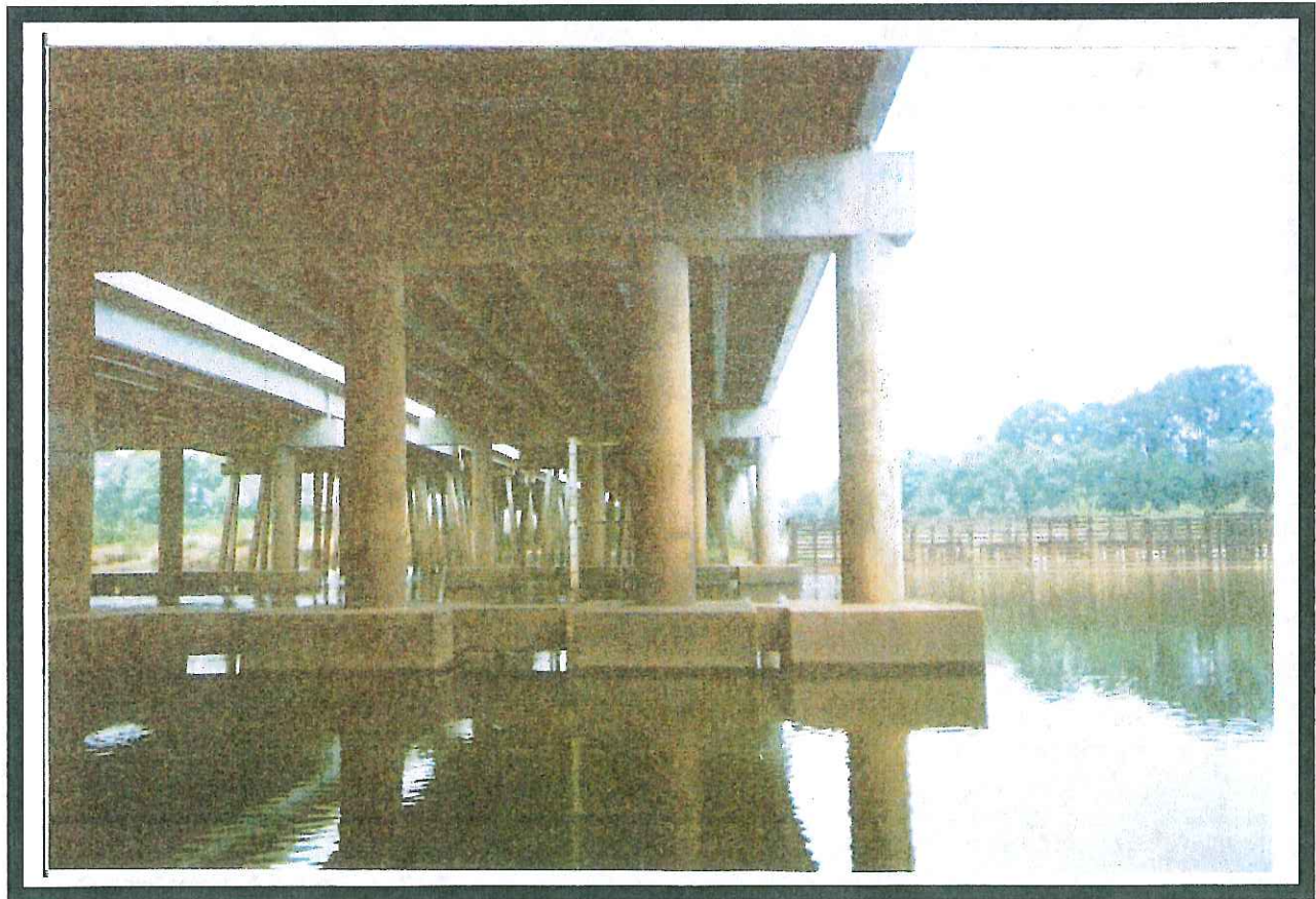
Figure 3. a. city water intake facility, b. Highway 25 bridge and revetment.
