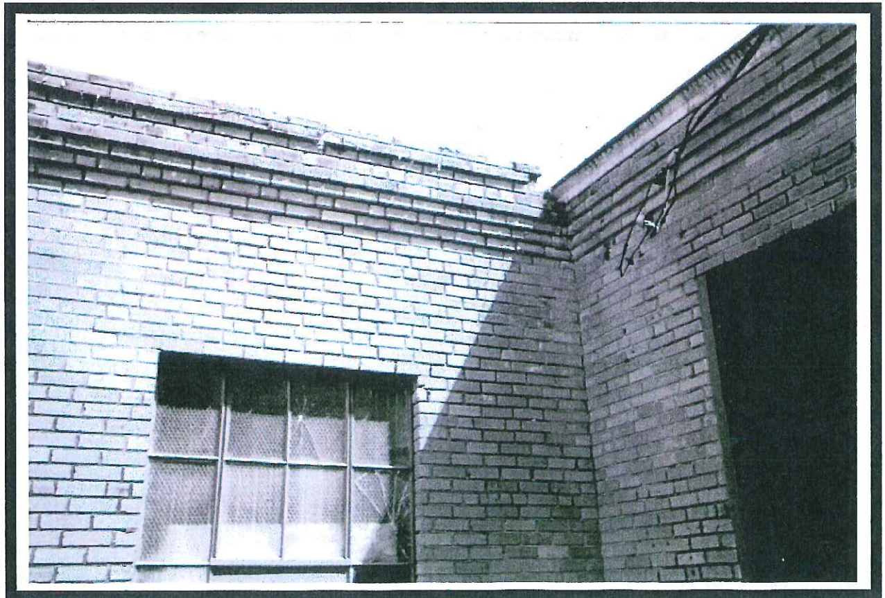
Figure 276. City Engineer Office; a. view west; b. cornice detail
