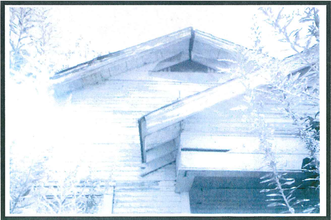
Figure 287. Farrish Street 532; a. porch detail windows; b. porch detail and eaves.
