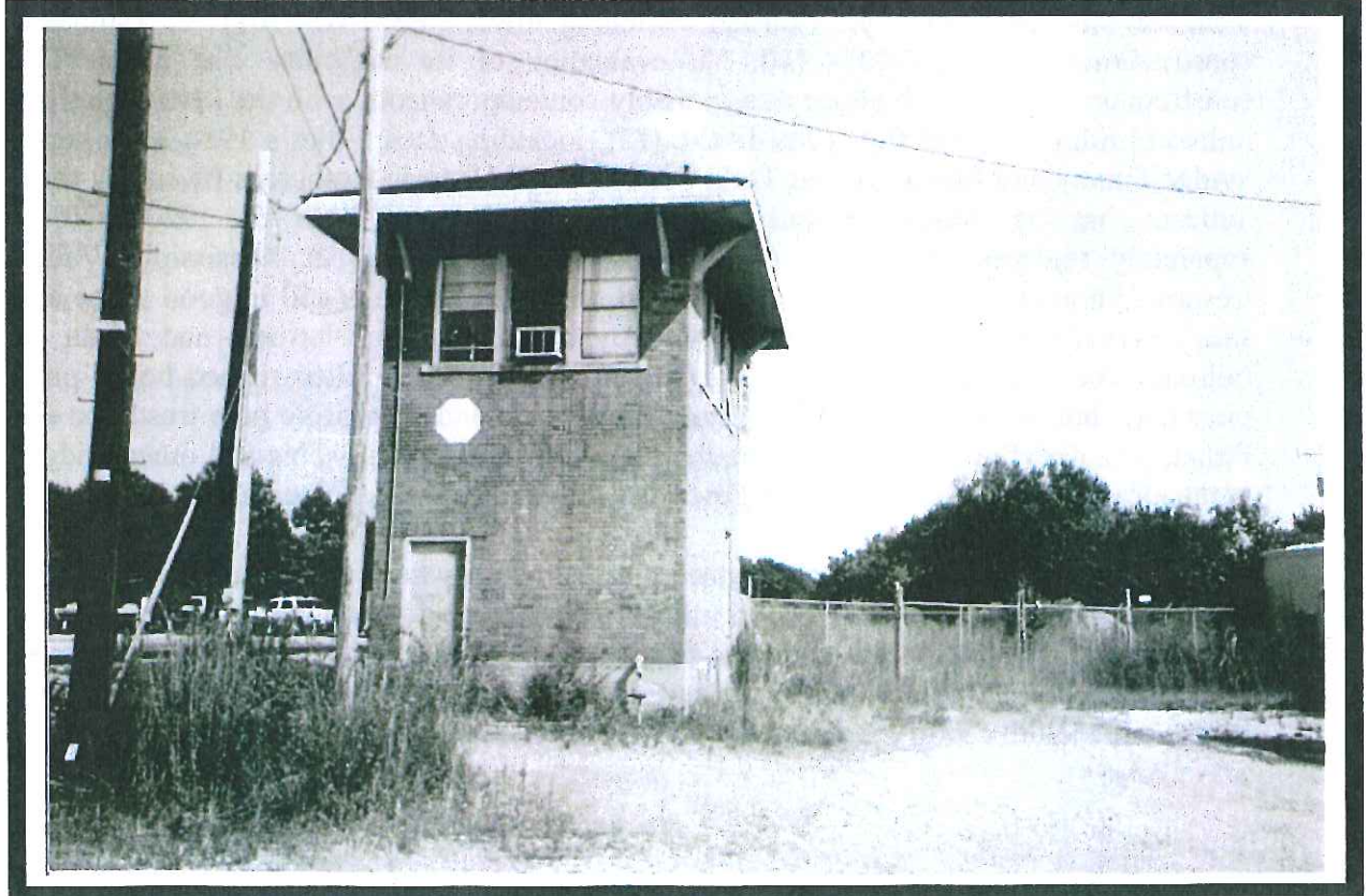
Figure 280. Kansas City Southern Switch House
