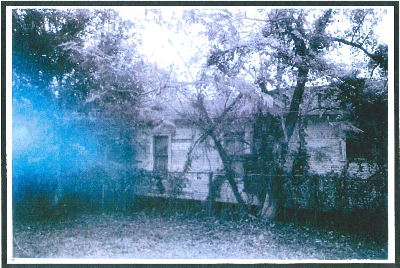
Figure 286. Farrish Street 532; a. façade; b. north side.
