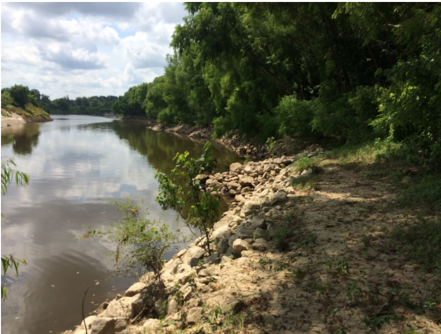
Picture 12 – Rip Rap Area along Bank of Pearl River
