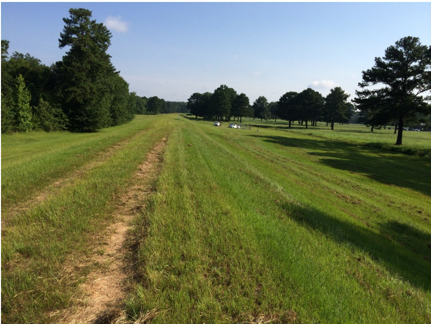
Picture 6 – Levee looking North
